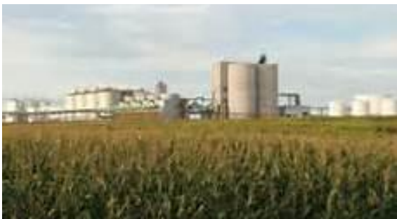
Valero Ethanol Plant – Industrial use located just outside of Hartley city limits
