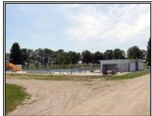
Photo of municipal swimming pool
